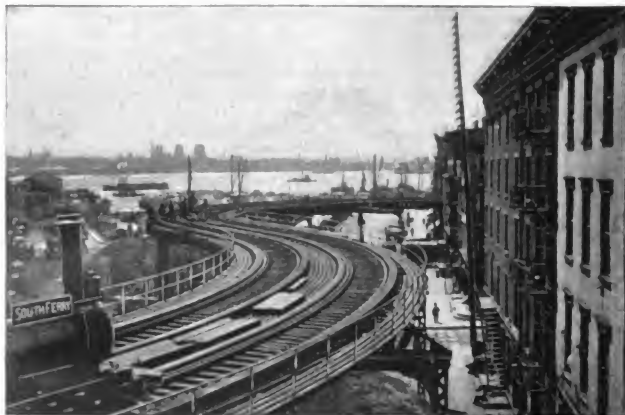
ELEVATED RAILROAD NEAR COENTIES SLIP, EAST RIVER.
